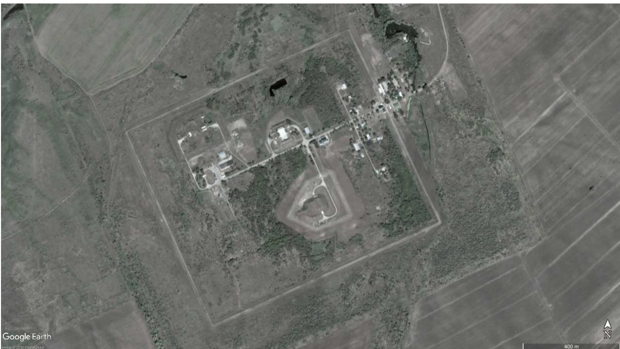
Figure A4. Base-level storage facility at Engels air base
